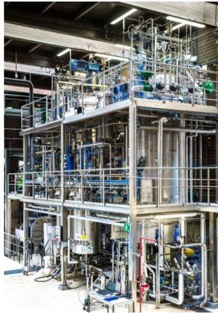
Figure 15: Pilot-scale 15 m 3 fermentation bioreactors for TAG production at BBEPP.
